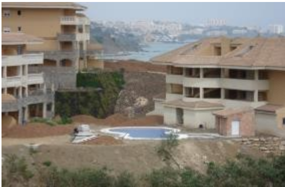
Construction site (Malaga, Spain). Credits: M. Palacios
