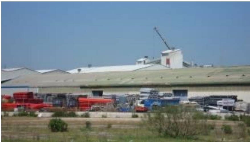
Industrial site (Madrid, Spain). Credits: M. Palacios
