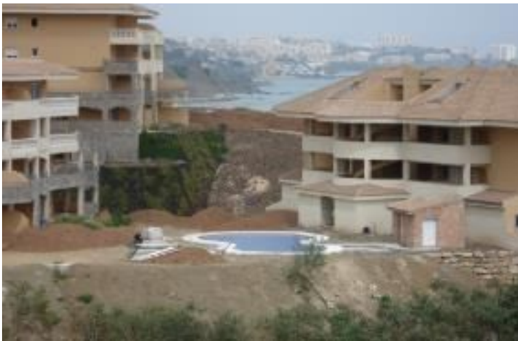
Construction site (Malaga, Spain). Credits: M. Palacios
