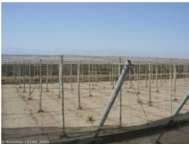
Greenhouses structure in Almeria (Andalusia, Spain). Credit: Eurostat Lucas 2009.
