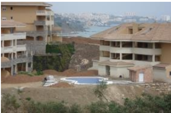
Construction site (Malaga, Spain). Credits: M. Palacios
