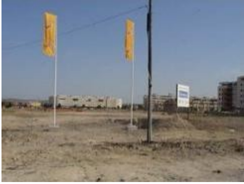
Construction site (Cadiz, Spain). Credits: M. Palacios
